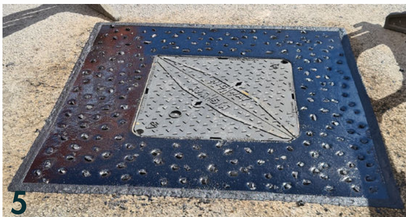
5 Finally, overbanding is applied.
