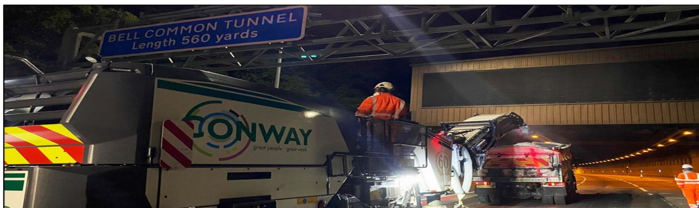
Image 5 – CPS M25 Bell Common Tunnel Resurfacing Scheme
